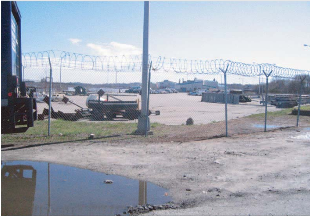
Homeport Site Development Parcel A: View facing south towards existing Homeport Site
