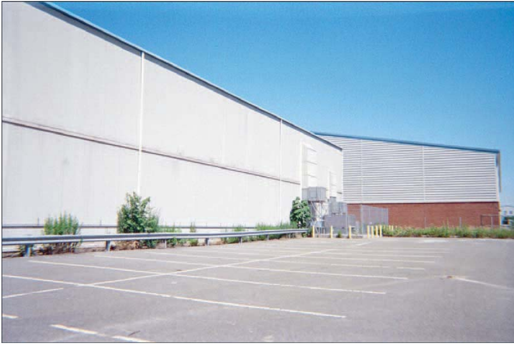
Homeport Site Development Parcel B4: View facing north towards existing Homeport Site Building 2.
