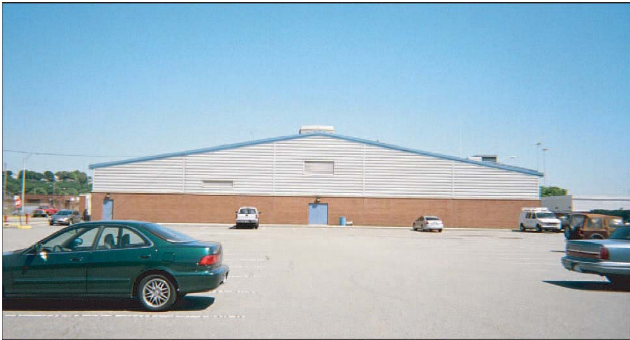
Homeport Site Development Parcel B3: View facing north towards existing Homeport Site Building 3.
